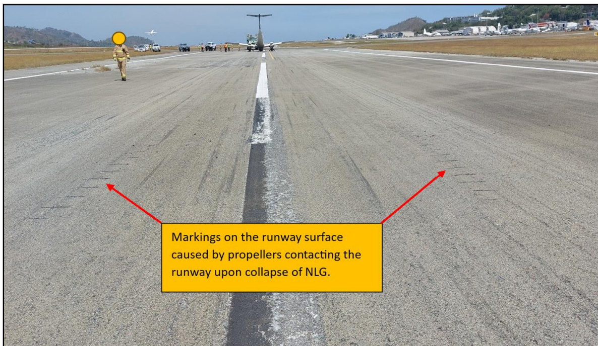
Figure 4:Runway Surface Markings-14R.
