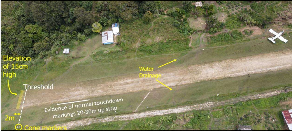
Figure 7: Tekin Airstrip with indications of onsite observation
