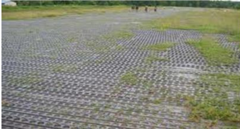
Figure 2: Steel Marsden matting 4
