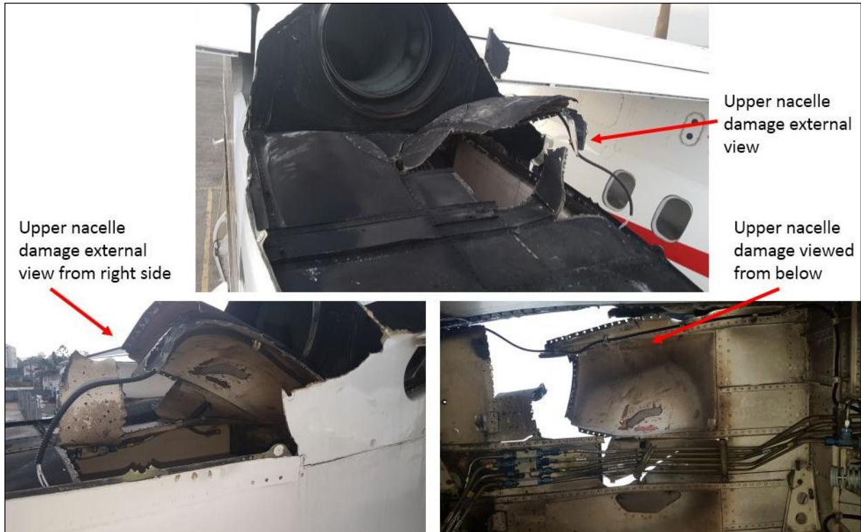
Figure 3: Damage area left nacelle
