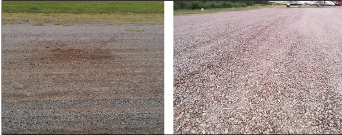
Figure 10: Bulolo Airstrip Surface Source: LinkPNG- Facility Inspection Report
